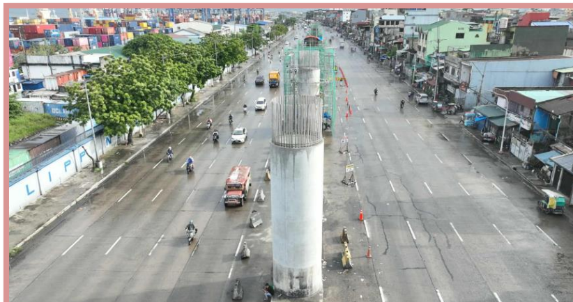
SP-49: Casted column up to 2 nd lift
