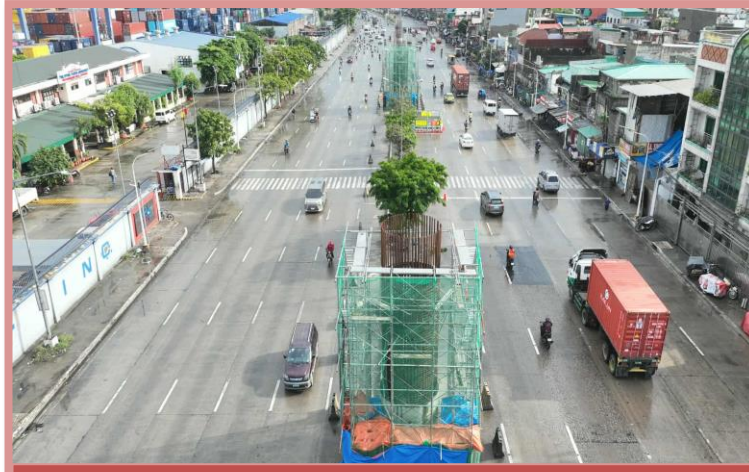
SP-51: Casted column up to 2 nd lift
