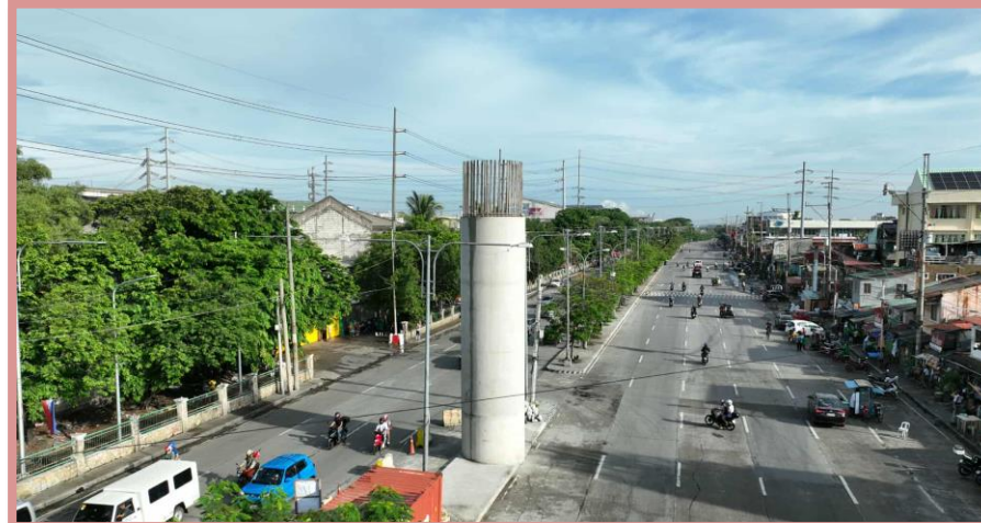
NP-14: Casted column up to 3rd lift
