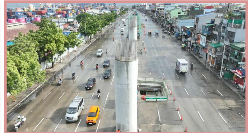
SP-48: Casted column up to 2 nd lift
