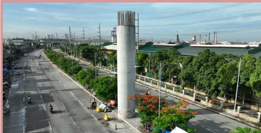
NP-10: Casted column up to 2 nd lift
