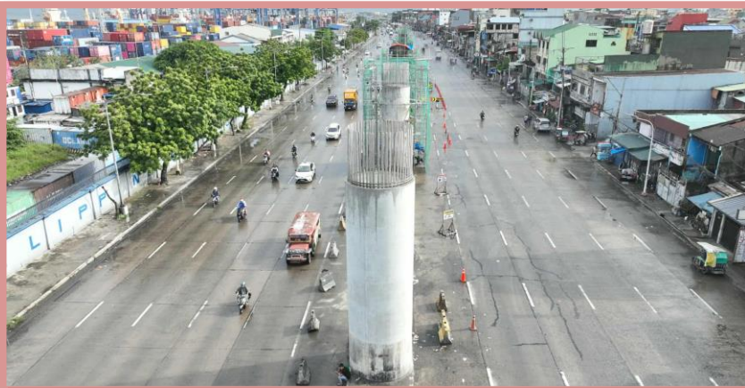
SP-50: Casted column up to 3 rd lift
